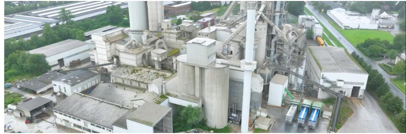
Phoenix Zementwerke Contract: CEBO° Pilot Campaign Status: completed Industry: Cement Delivery: 2023 Location: Beckum, Germany Duration: 10 months Capture capacity:  $25.3 \text{ t CO}_2$ Capture efficiency: 90-95%
